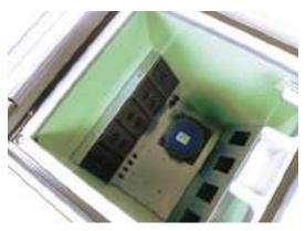
Convention Center Floor Box wiring compartment.
