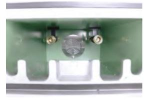
Convention Center Floor Box water and compressed air compartment.
