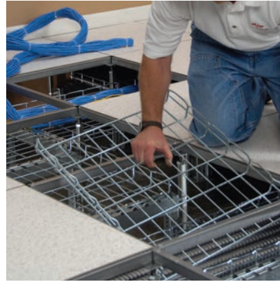
Place 2' tray sections in position.
