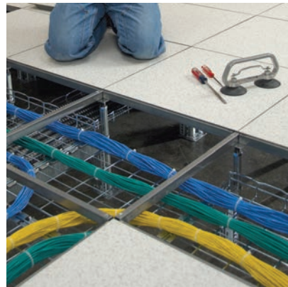
Use a UFT90KIT for corners, tees, and junctions. Secure with tray clips.
